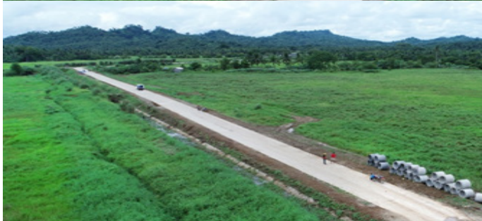
Aerial shot of the recently-completed Bulao-Santa Fe Farm-to-Market (FMR) road.
